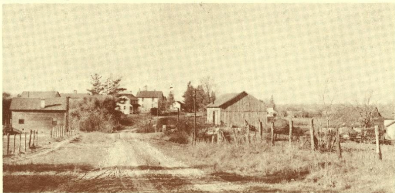
Muehlbauer Blacksmith Shop on the right. The building on the left was the cheese factory.
